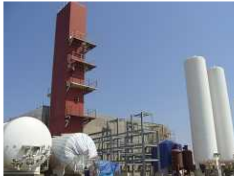
Picture: Air separation plant under construction in Vietnam (Hanoi)
