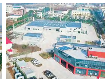
View of an electronic materials gases production facility in China
