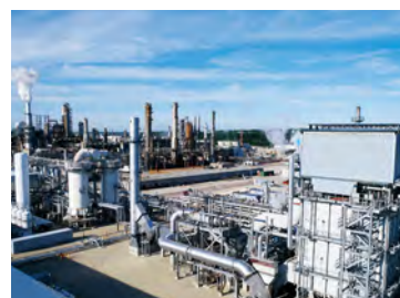
HyCO production facility
