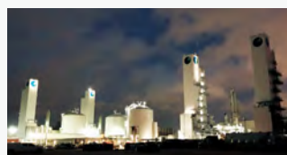
On-site plant method ASU in operation at Westlake Chemical (Texas)
