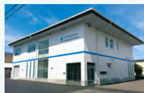
Exterior view of the TNSC Technical Academy
