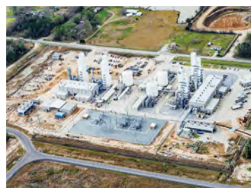
Westlake on-site piped gas facility
