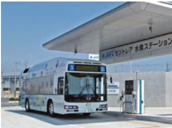
Hydrogen filling station
