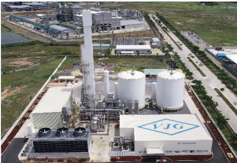
Phu My 3 air separation unit installed in an industrial park (Completed September 2019)
