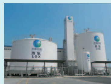
Air separation plant at Dalian Changxing Island Taiyo Nippon Sanso Gas (China)
