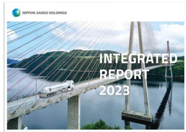
NSHD Integrated Report 2023 (Released on September 26, 2023.) Please jump to the access webpage.> Link
