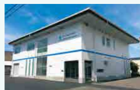
Exterior view of the TNSC Technical Academy
