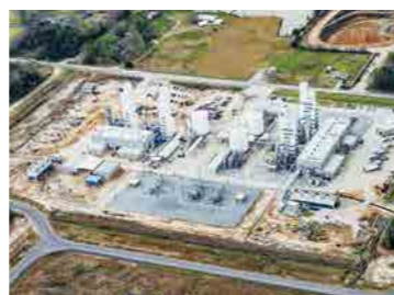
Westlake on-site piped gas facility
