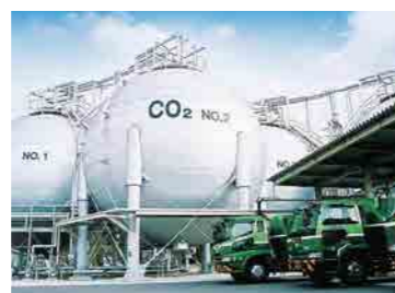
Nippon Ekitan Corporation carbon dioxide gas terminal
