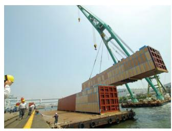
Large-scale air separation unit on its way to Sasol Chemicals (USA)
