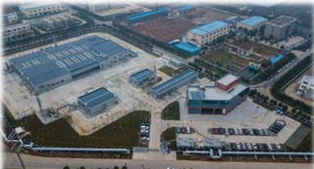
China: plane view of electronics material gases plant (1 st period)
