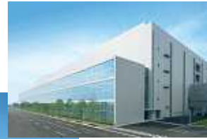
Thin-film solar cell plant
