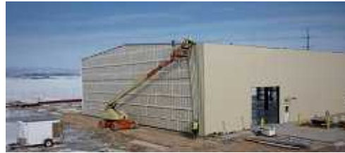
Picture: New plant under construction
