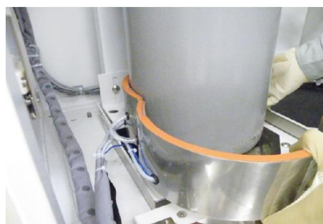
Installing NACS HEAT® on a 47-liter cylinder
