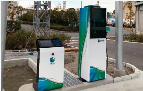
Hydrogen filling system at the Kawasaki-Mizue Business Base
