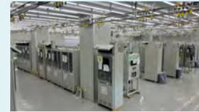
Equipment factory of TNET
